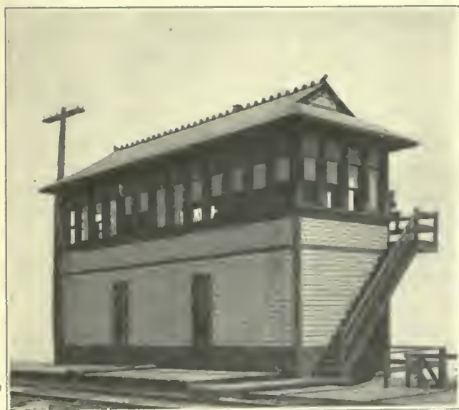
FIG. 291. INTERLOCKING PLANTS. 43d Street interlocking tower of the Illinois Central Railroad. This plant is typical of a number of mechanically operated interlockers throughout the Area of Investigation.
